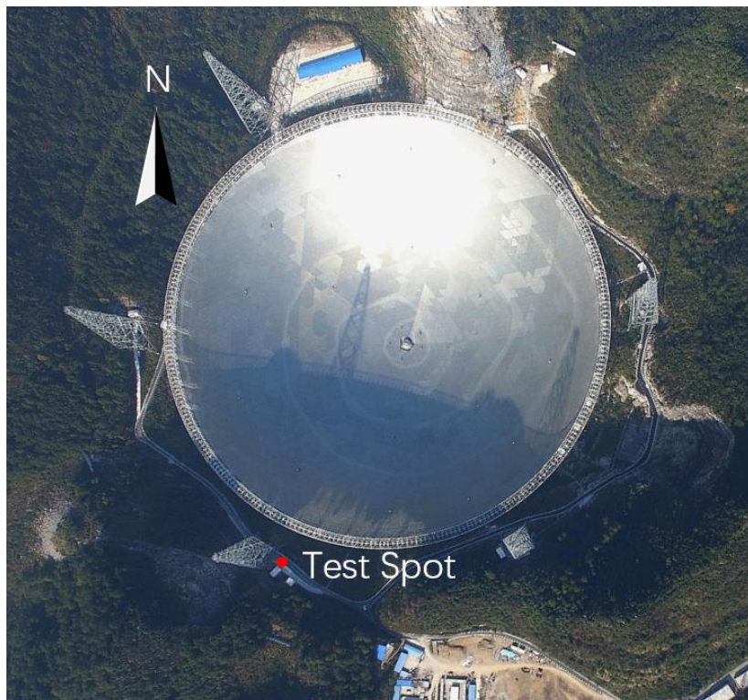
Fig.1 RFI test spot at the bottom of the 7H feed support tower.
